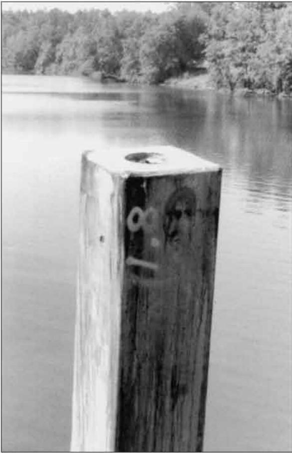
*An undamaged cement bridge pile after being driven using APS Hammer Cushion Pads. There was no need to trim the top, a costly and time consuming job. Also, the life of the APS Hammer Cushion Pad is longer so there is less time lost in changing pads.*
